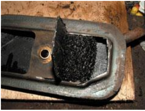
Remove and inspect the old breather gauze
